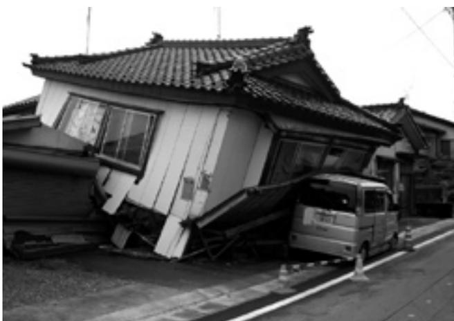
*A car supporting a house collapsed by the Niigata Earthquake*
